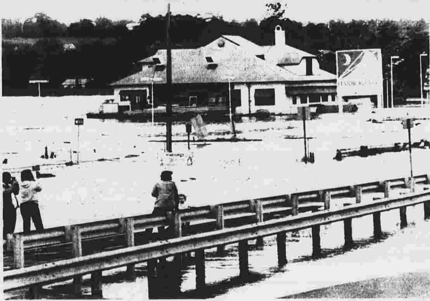
Friday, 24 hours before the Connecticut River is expected to crest in Middletown, water reaches the second floor of the Harbor Park restaurant and blocks
